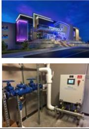
**GM Flint Assembly Plant: Hubbell Model EMV120-85-1.5SLA-A-XX Electric Tepid Water Heater**
