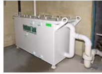
Elevator Sump Pump Interceptors
